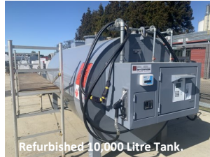
Refurbished 10,000 Litre Tank.
